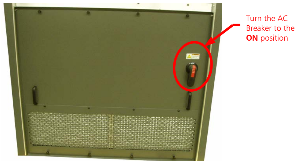
Figure 3-7: Turn AC Breaker to ON
