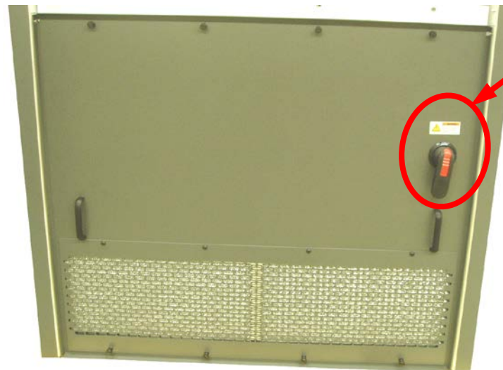
Figure 3-2: Turn AC Breaker to OFF
