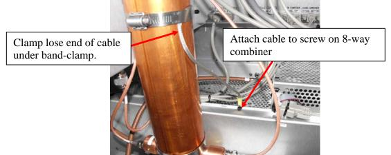
Figure 5. RFI Eliminator ground connection on FM-10S/703.
