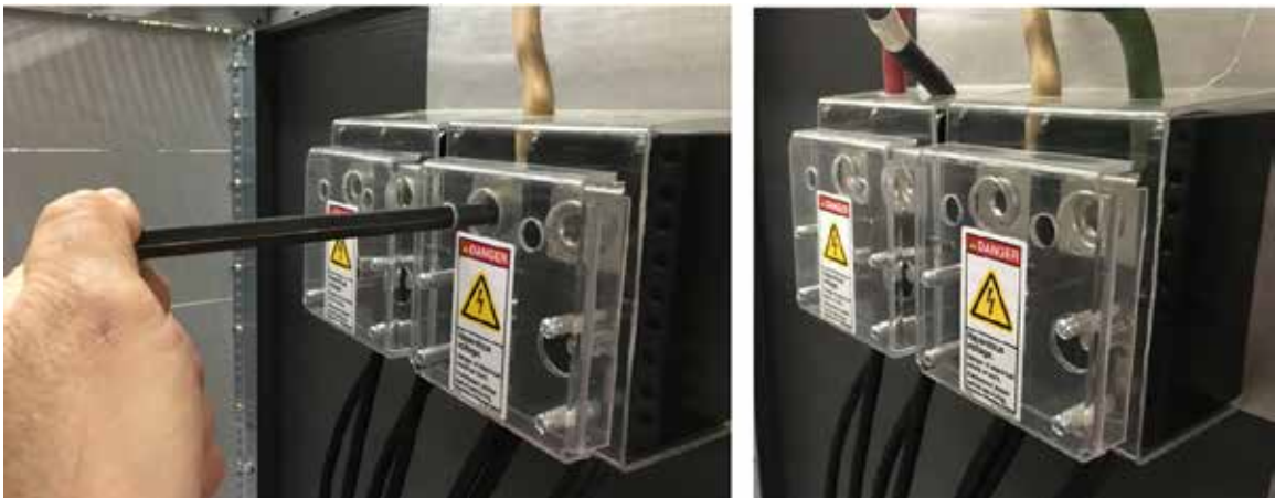
Figure 4 – STX 20 Main AC Terminal Block
